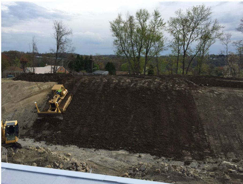
Spreading Topsoil
