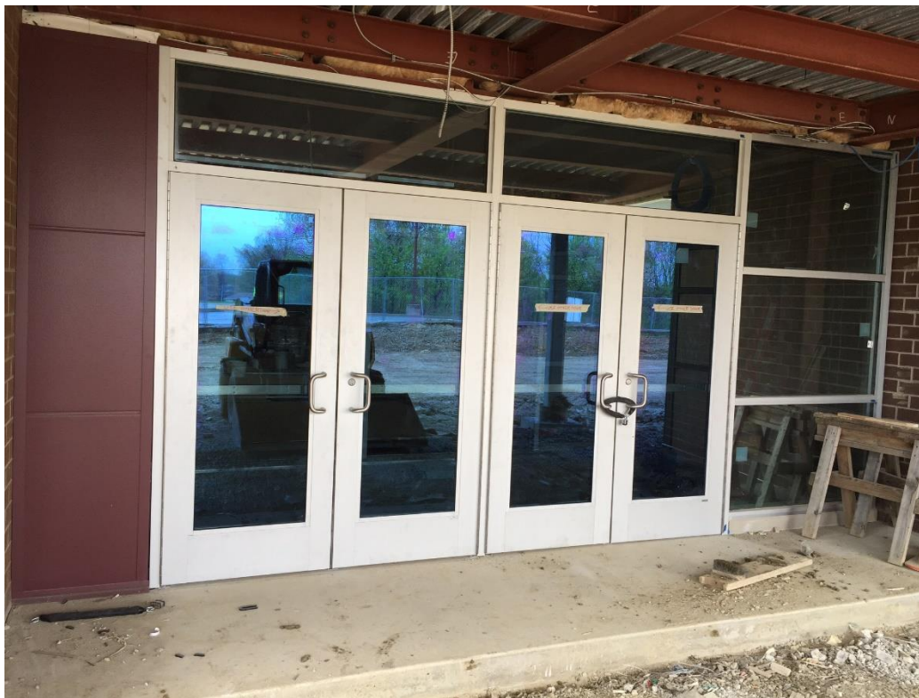
Area A Entrance Doors
